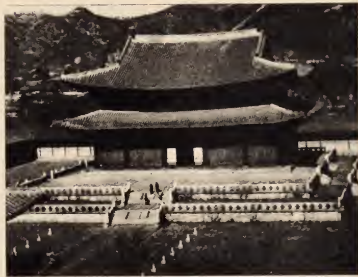
Administration Hall of Kyongbok Palace rebuilt in 1859
